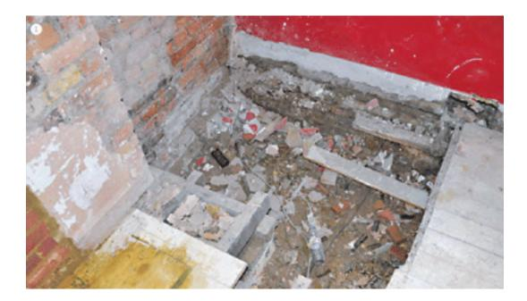
Figure 1: General builder?s rubble and arisings placed under the timber suspended floor following property refurbishments
