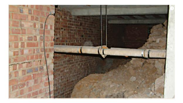
Figure 3: Deep void below a solid suspended floor full of earth and rubble that needed excavation to remove the threat of excessive dampness and resultant condensation. Water droplets were found to the underside of the solid floor, which did not have an impermeable vapour barrier
