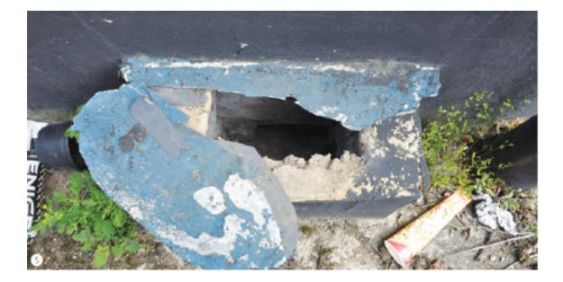
The low level through-wall air vent was shrouded with a half brick thick wall because the external ground level is far too high above the location of the air vent. A slate had been placed over the top of the brickwork to prevent rainwater induction. Another vent to the outer brick created a periscopic ventilation system. The failed slate top resulted in substantial rain water penetration through to the internal suspended timber floor
