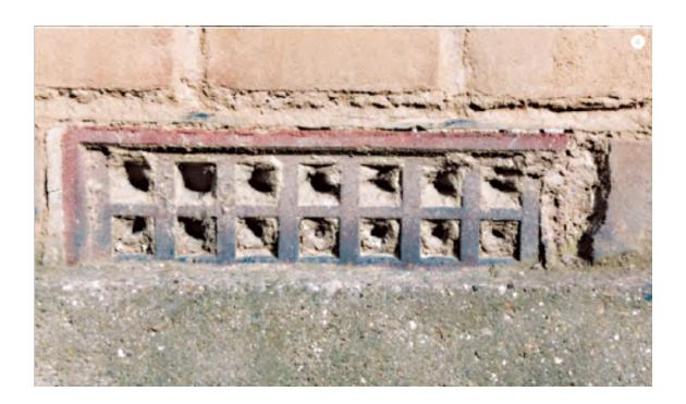
Blocked low level through-wall air vent. The physical damp proof course is just above the vent. The abutting solid concrete patio is in contact with the bottom edge of the vent, sufficient for rainwater to penetrate through the air grill. Rain splash from the hard external surface will introduce dampness into the solid masonry wall above the height of the horizontal damp proof course
