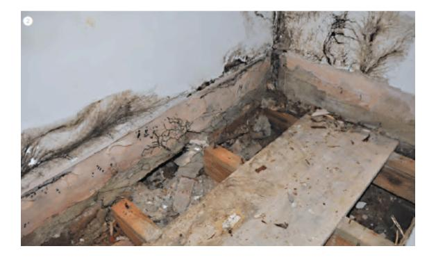
Figure 2: Blocked external low level through-wall vents to the sub-floor. The resultant increased moisture activity led to an outbreak of the dry rot fungus *serpula lacrymans*
