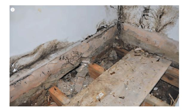
Figure 2: Blocked external low level through-wall vents to the sub-floor. The resultant increased moisture activity led to an outbreak of the dry rot fungus *serpula lacrymans*
