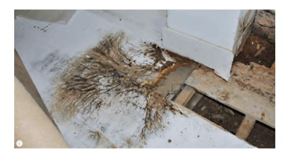
Timber suspended floor and solid fire hearth that had also been over-boarded with timber plywood panels. The dry rot outbreak was due to high abutting ground levels, which had blocked the low level through-wall air vents, and low level dampness penetration through the solid external walls; the sub-floor void was very shallow and a high water table also helped produce the ideal environment
