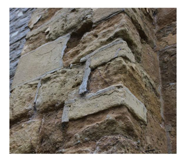
Figure 1: Severe erosion of soft sandstone blocks on an ancient building following inappropriate repointing with OPC mortar
